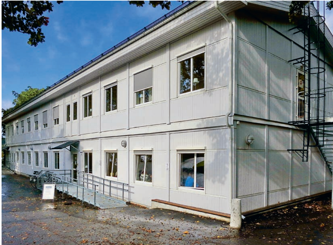
The integration of the teachers' training in 2008 implied a severe scarcity of offices and classrooms for the University. Here a temporary pavilion for teachers and researchers at the Department. (Photo: Mats Danielson)
