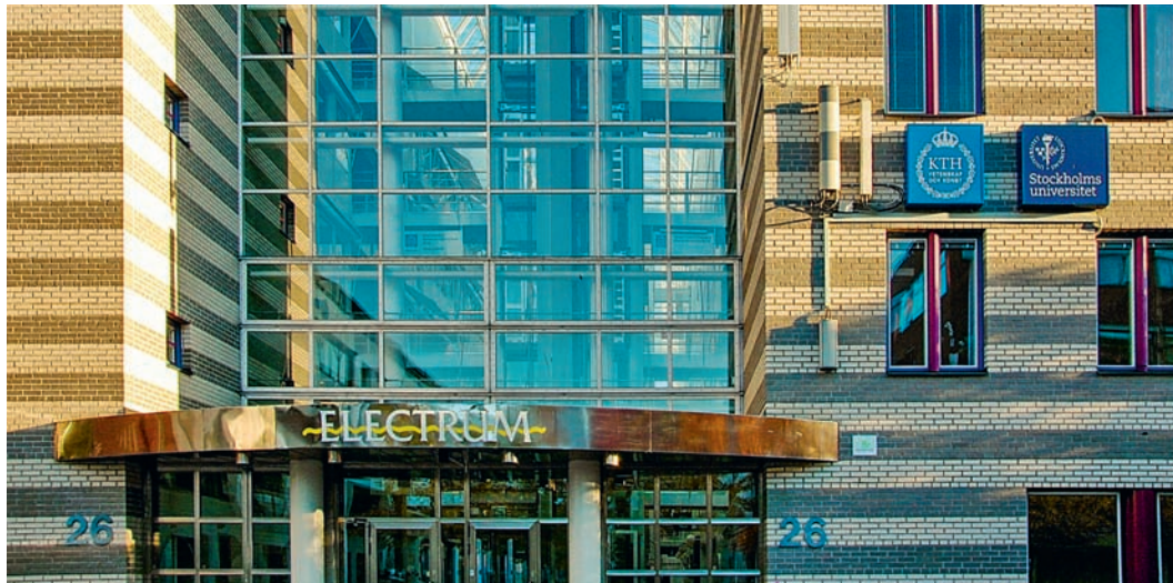
The Electrum building in Kista, home of the Department between the years 1990 and 2001. (Photo: Mats Danielson)
