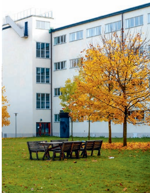
The Sveaplan building from behind.
